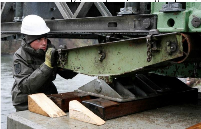
Figure 12: Corrective Maintenance – Temporary repair of a bridge (Bundesheer, Moser, 2009)
